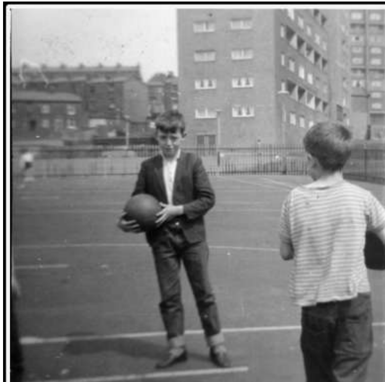
St Peters School playground with Mazzini maisonettes in the background
